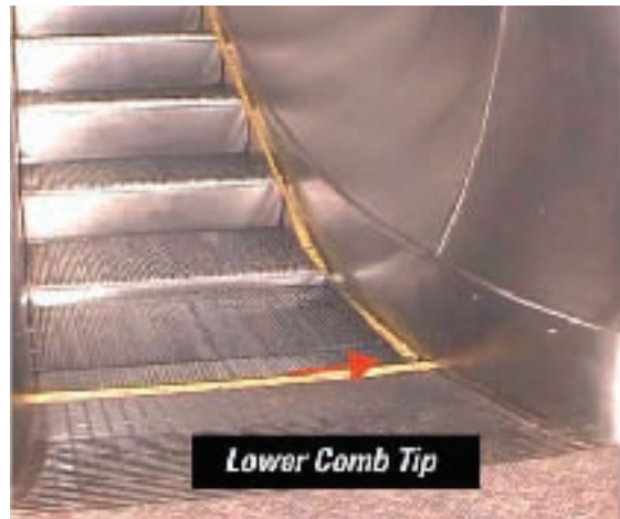
Bottom landing: Lower Comb Tip
